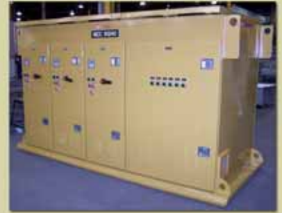
Portable 600 V Mine Motor Starter
